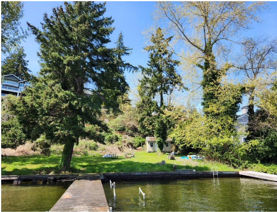
Photo 1. Existing shoreline conditions, taken from southern dock facing west.
